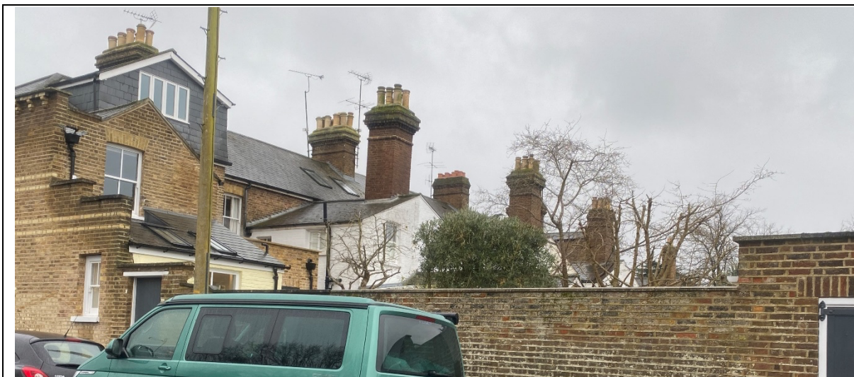
Figure 20 Roof lights to the rear of the south terrace of The Mount
