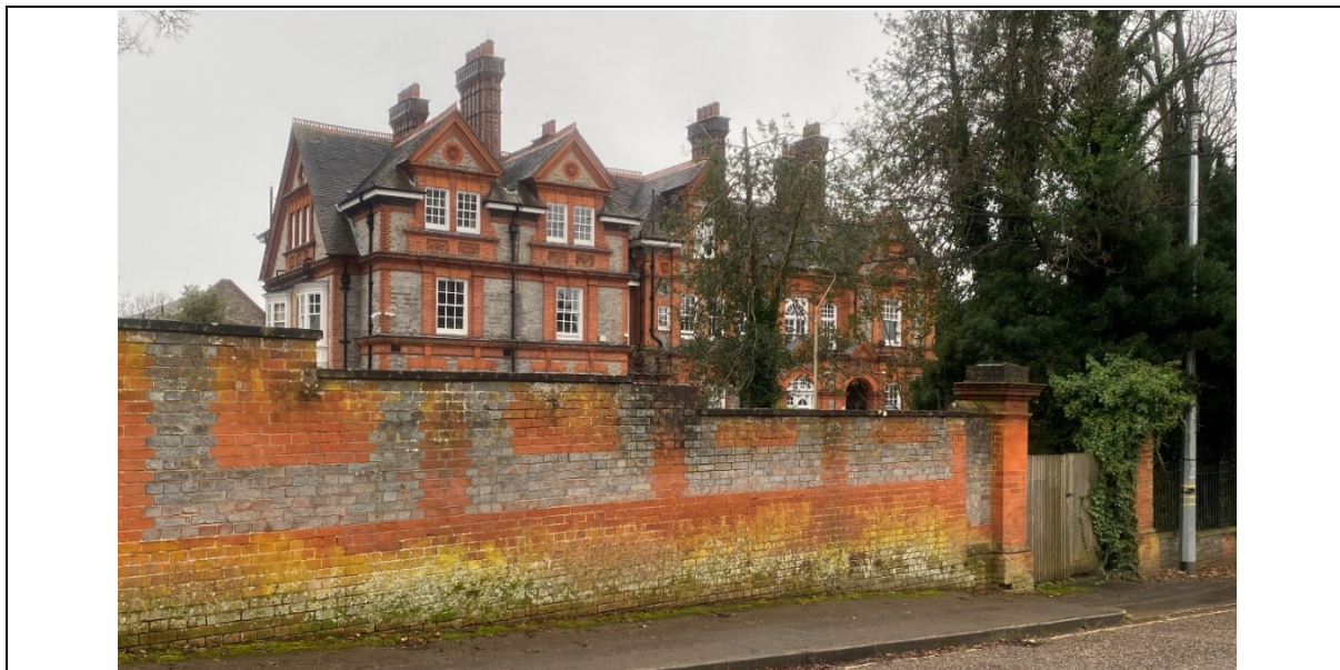
Figure 21 View of the east elevation of Hillside from Lower Mount (Image Claire Truman)
