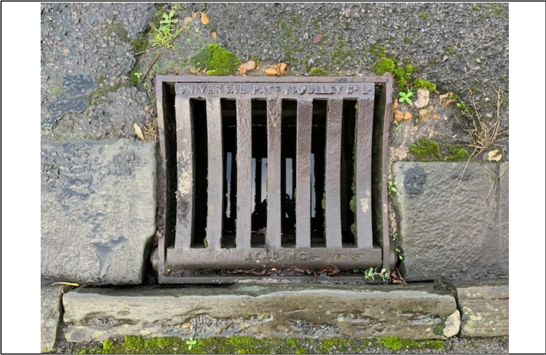
Figure 13 Universal Patent Pulley Co drain set within 'Caithness Flagstone Series' gutter and kerb stones (Image Evelyn Williams)
