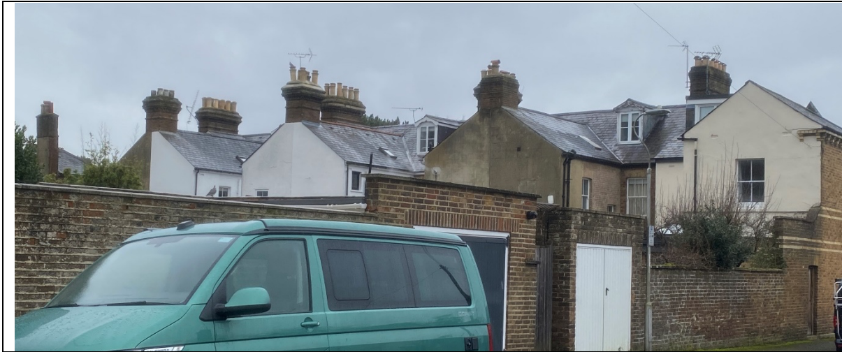
Figure 19 Original dormer windows to the rear of the north terrace of The Mount
