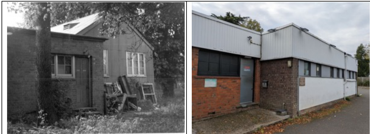
Figure 36 The north side of the Progress Theatre. (Left) stage door c1950 and (right) today when the corrugated iron club hall has been obscured by later extensions. Images courtesy Progress Theatre
