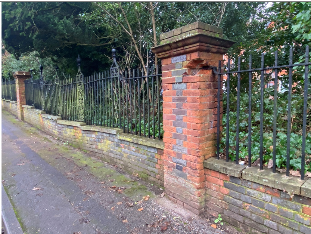
Figure 20 The brick piers and railings to Hillside are falling into disrepair – view along Lower Mount ( image Claire Truman )
